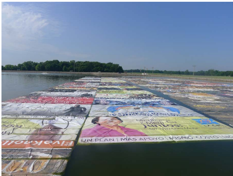
Fabricated Covers on Lagoon 2
