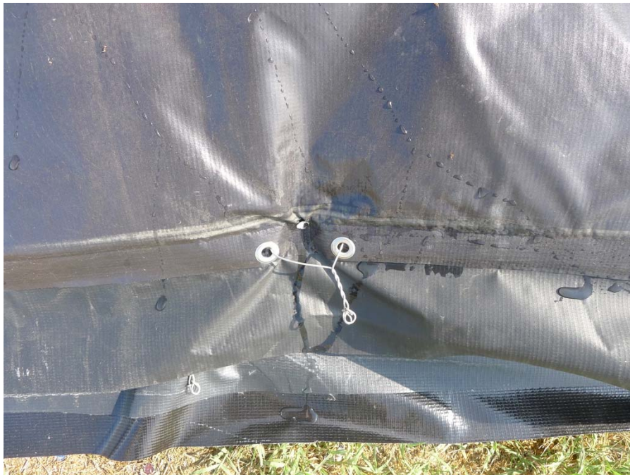
Detail of Connector for Attaching and Connecting Panels
