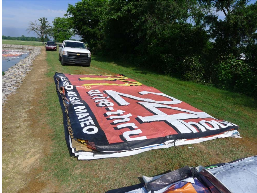
Covers Stacked for Deployment onto Lagoon 2
